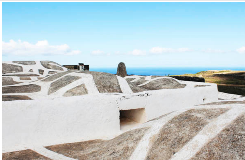
Dammusi with undulating roof to collect rainwater, copyright A Johansson
